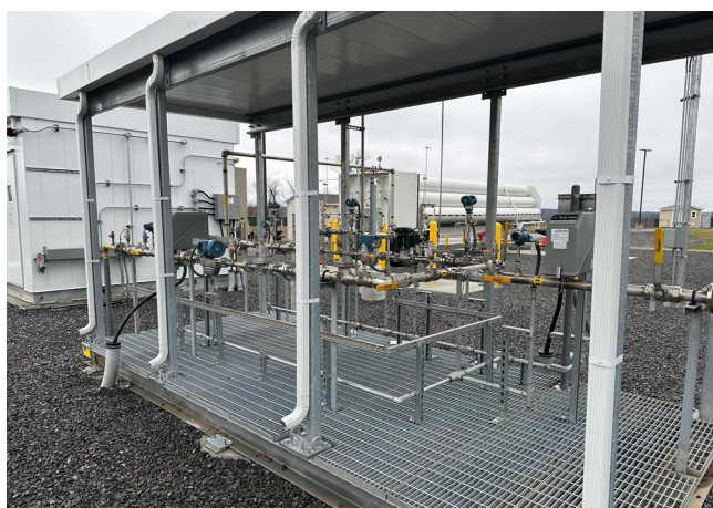
Hydrogen Blending Skid in Monaca, PA
