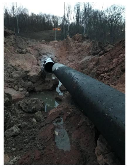
Figure E-5 In-service failure of a girth weld with weld strength undermatching
