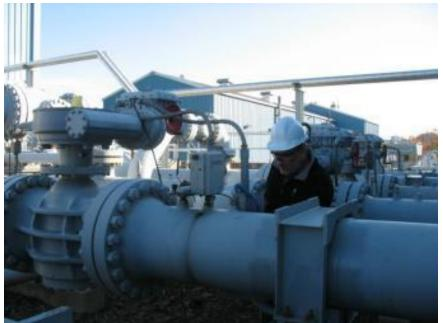
Figure 6. Example unit isolation valve.
