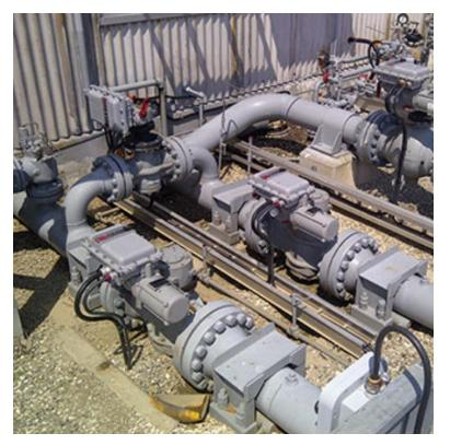
Figure 8. Example compressor unit isolation valve system for suction, discharge and bypass.
