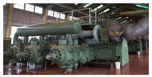
Figure 3. Integral reciprocating compressors.
