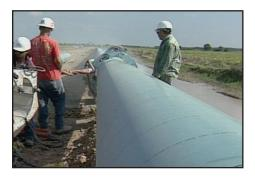
the type of coating used, the purpose is the same: prevent external corrosion by prohibiting moisture from coming into direct contact with the metal.
