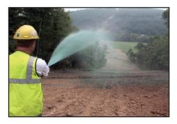
to divert water. The restoration crew also installs riprap, consisting of stones or timbers, along streams and wetlands to stabilize soils. As a final measure, the crew may plant seed and mulch the construction right-of-way, to ensure that foliage and grassland are restored as close as possible to their original condition.
