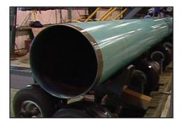
Prior to lowering the pipe into the trench, the coating of the entire pipeline is inspected to ensure it is free of defects.
