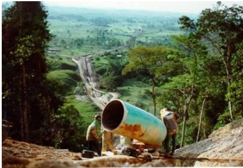
Figure 1. Induction bend being used during construction of a cross-country pipeline
