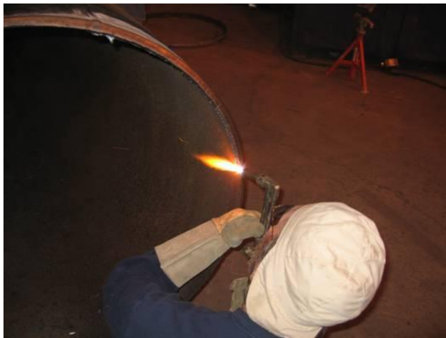
Figure 37. Flame cutting of transition on segmented bend
