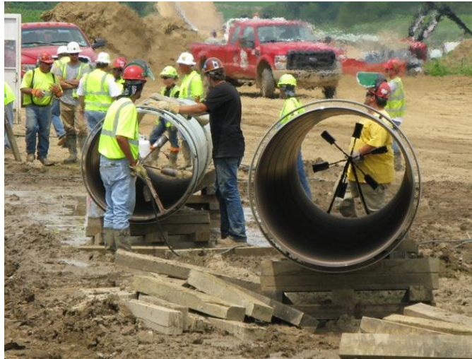
Figure B3. Preheating during pipeline construction activities
