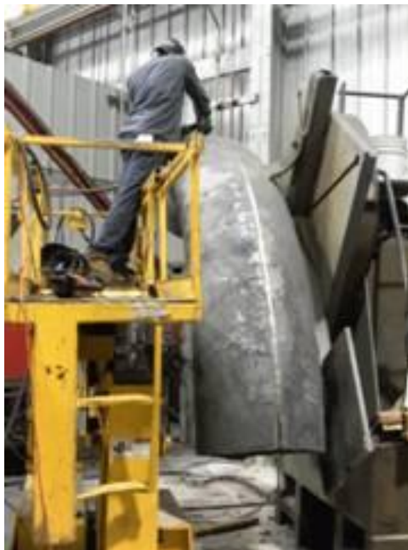
Figure 8. Seam welding using submerged arc welding
