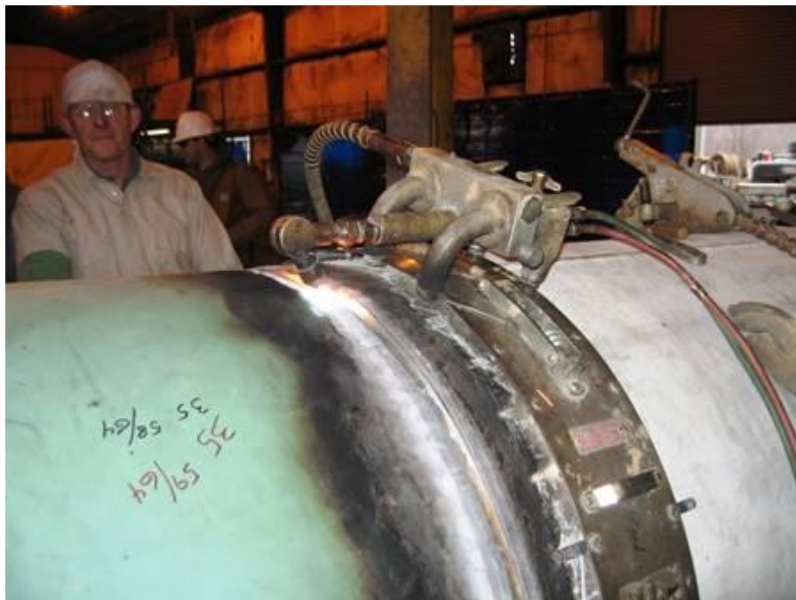
Figure 34. Flame cutting bevel on segmented induction bend from straight pipe side
