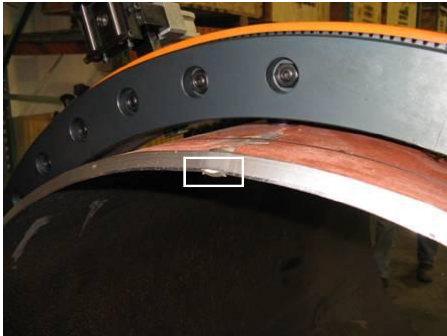
Figure 55. Completed weld bevel
