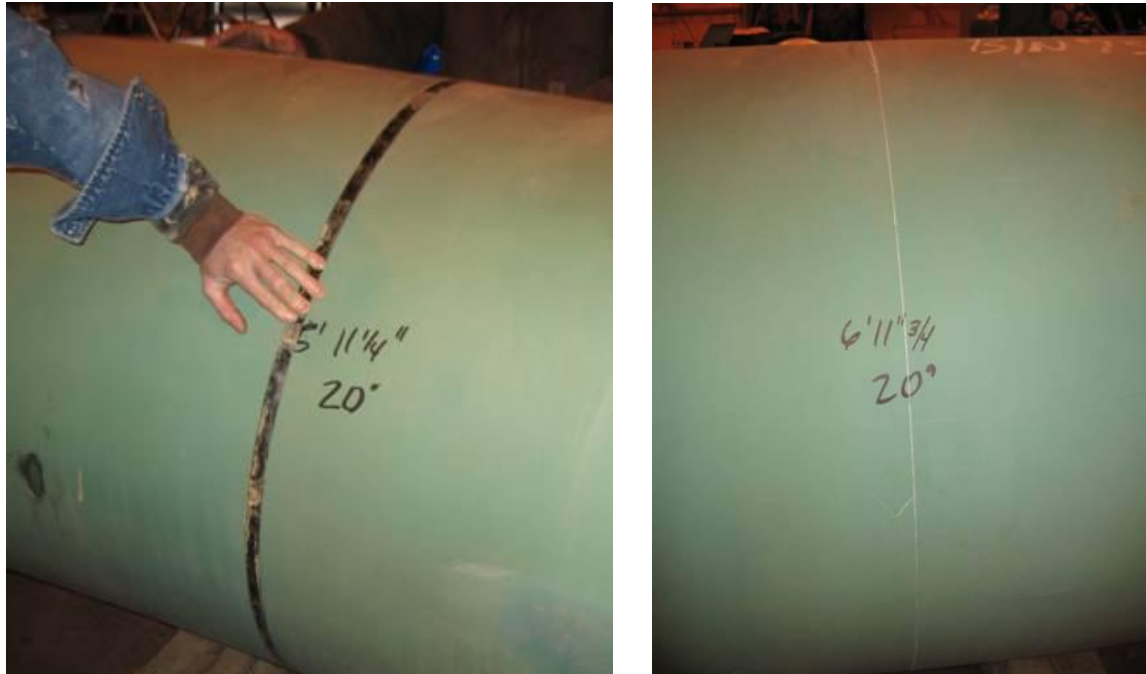
Figure 26. 3/4 inch wide steel strap and marked line for rough cutting
