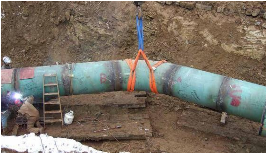
Figure 86. Segmented induction bend with double pups
