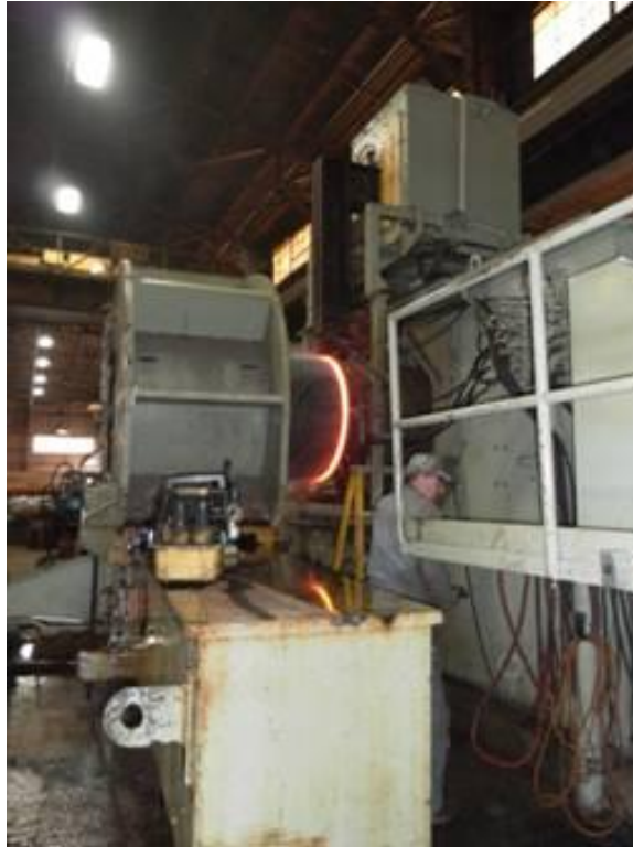
Figure 3. Heated portion of pipe material during induction bending process
