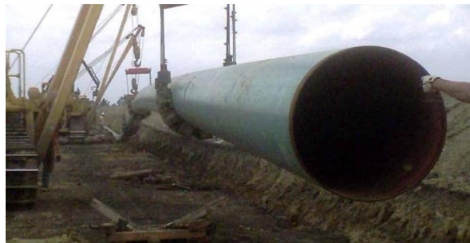
Figure B4. Pipeline lifting and lowering-in
