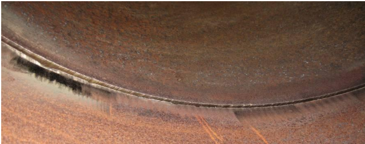
Figure 35. Fit-up of segmented bend to pipe pup section prior to transitioning
