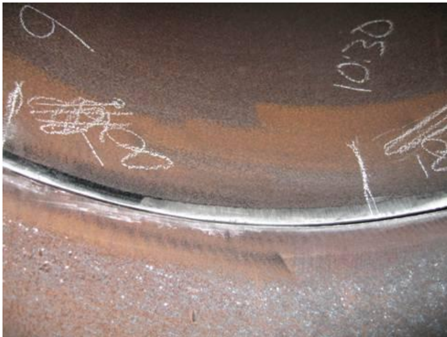
Figure 42. Fit-up of segmented bend to pipe pup section after transitioning
