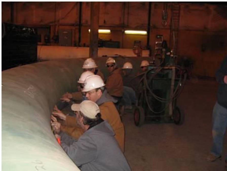
Figure 25. Measuring along intrados
