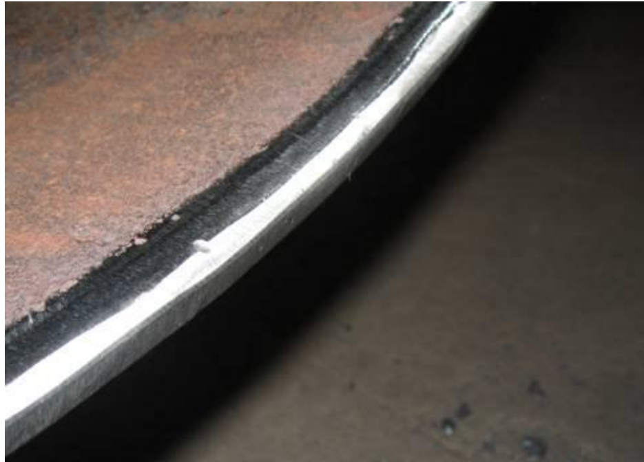
Figure 38. Transition on segmented bend after grinding
