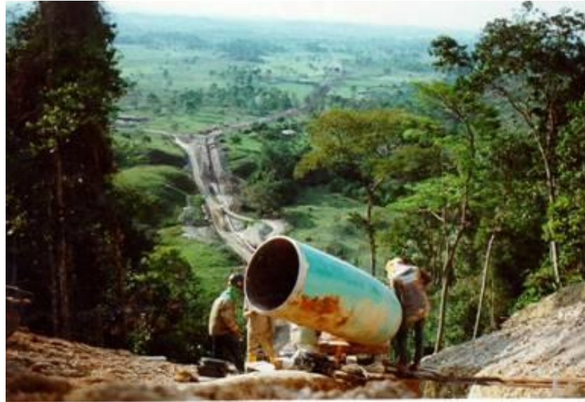
Figure 1. INDUCTION BEND BEING USED DURING CONSTRUCTION OF A CROSS-COUNTRY PIPELINE
